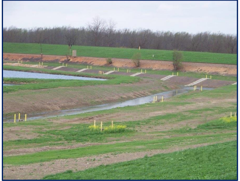
Completed Relief Wells Project, MO.
